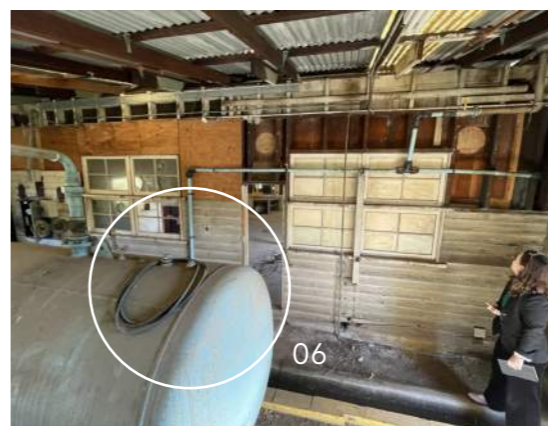
06 tank to be preserved
