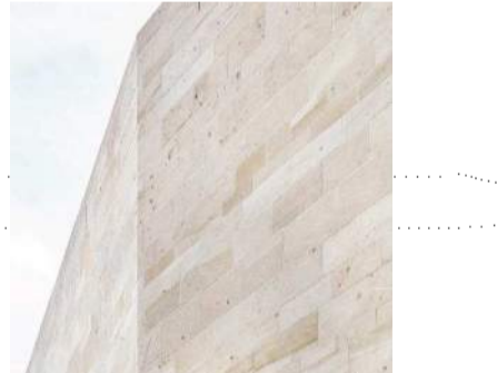
07 RETAINING WALL - TBC
