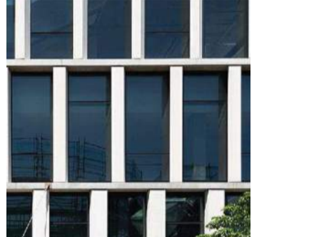
05 CONCRETE EXPOSED SLAB EDGE
