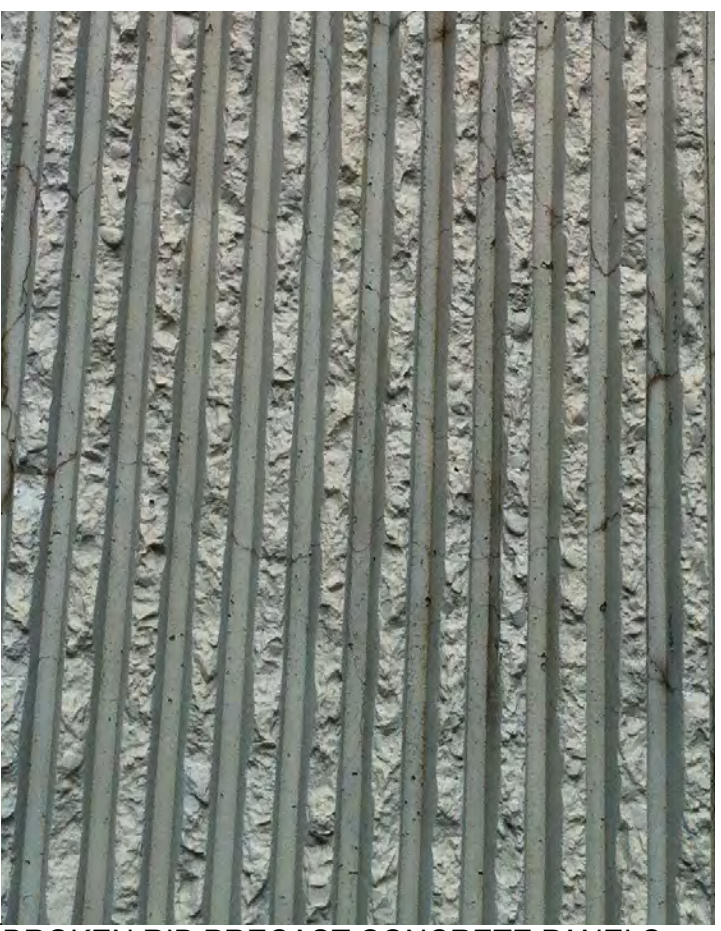
BROKEN RIB PRECAST CONCRETE PANELS
