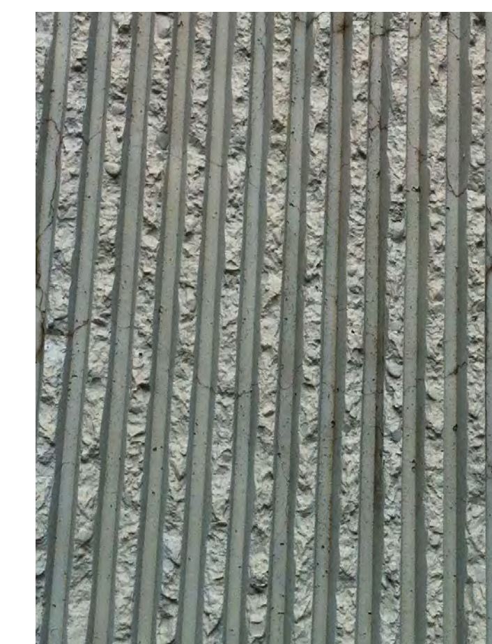
BROKEN RIB PRECAST CONCRETE PANELS
